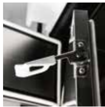
▲ Outer door latch with padlock panel
